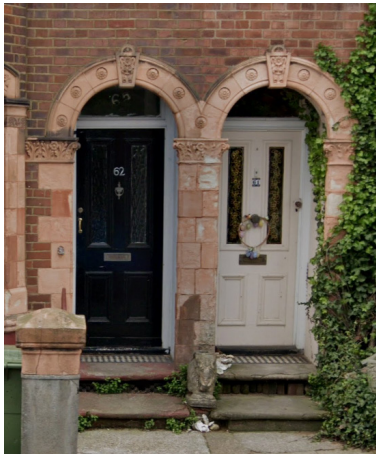
Recessed entrance with tiles
