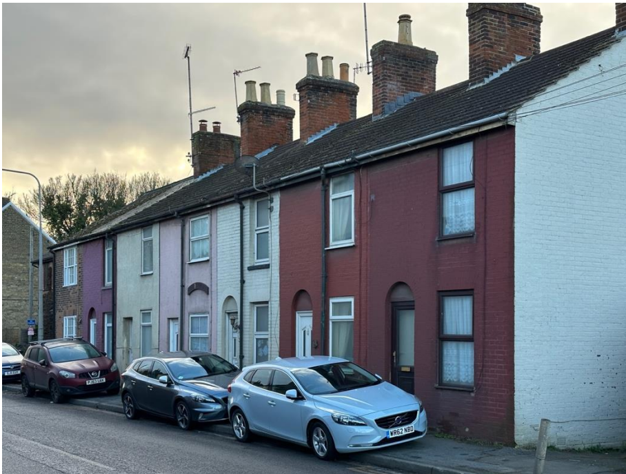
Terraced properties to the south of Canterbury Road.
