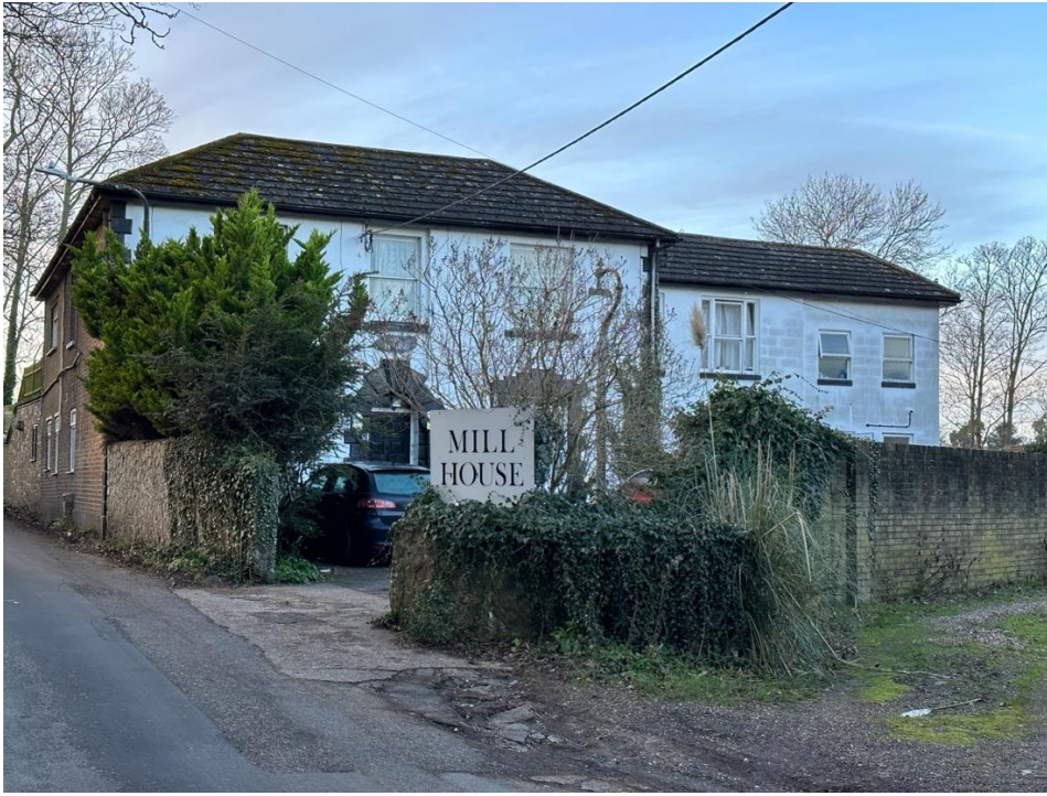
Mill House: The property is side-on to the road.
